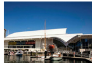
Commissioning Plan | O&M Manuals: Australian National Maritime Museum
