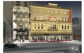
Electrical Services O&M Manual | Her Majesty's Theatre Renewal Project
