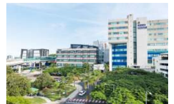
Fire O&M Manuals | Royal Brisbane and Women's Hospital (RBWH) Fire Detection Upgrade Building 39, 40 & 41, QLD
