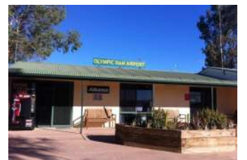
Mechanical O&M Manual and Commissioning Plan | Olympic Dam Airport Upgrade, SA
