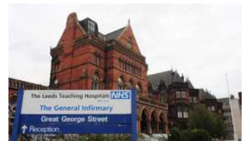
Mechanical O&M Manual | Leeds General Infirmary CAT Unit, UK
