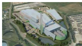
Viridor Recycling Plant, Polymer 2 Administrative Office Fitout
