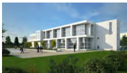
Advanced Technology Building Dundalk, Ireland
